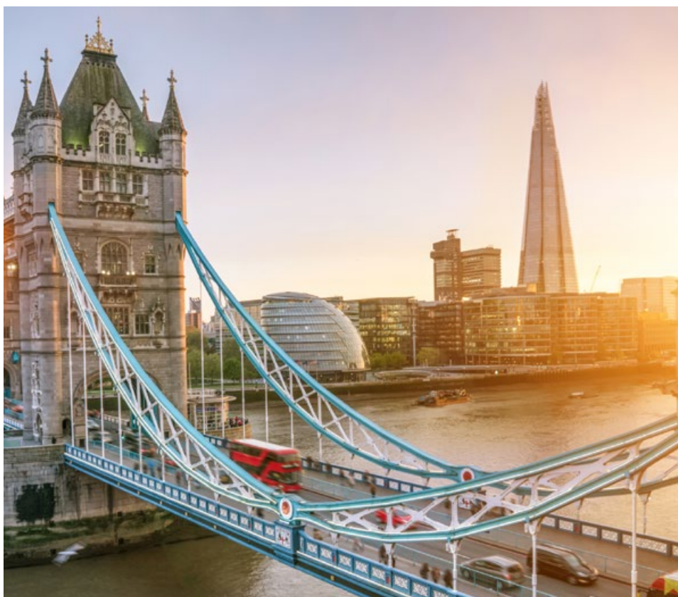
Tower Bridge, with views of City Hall and The Shard
